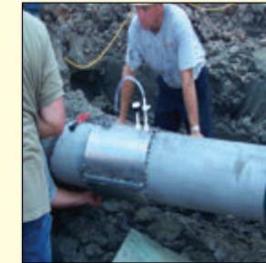
6) install steel mold
