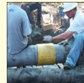
12) pipe repair complete
